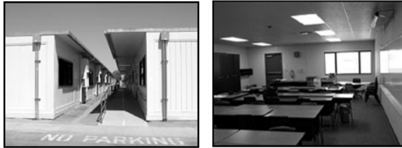
Figure 6. Portables: 24' x 40' Modular Classrooms with Exterior Entrances, Typically Lined Up in North or South Facing Rows, With 4' X 8' Windows on Both Narrow Ends
